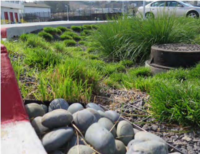
Bioretention in an industrial area of San Francisco. Photo: Krystal Zamora
